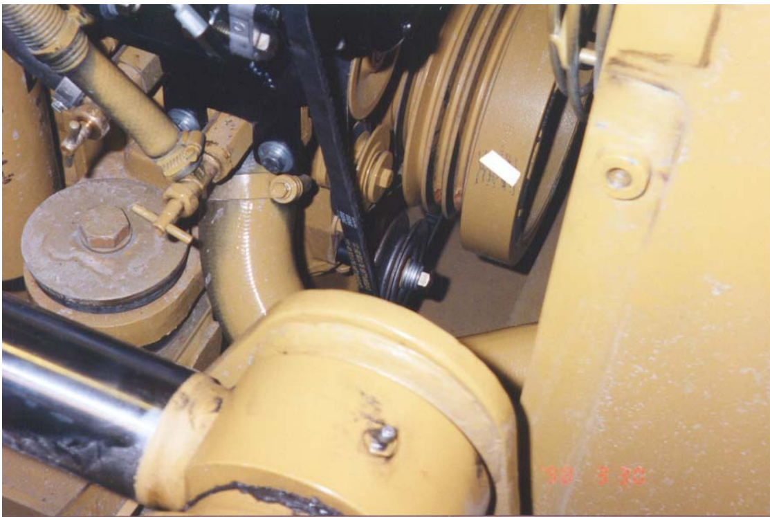
Compressor mount and drive with idler pulley.
