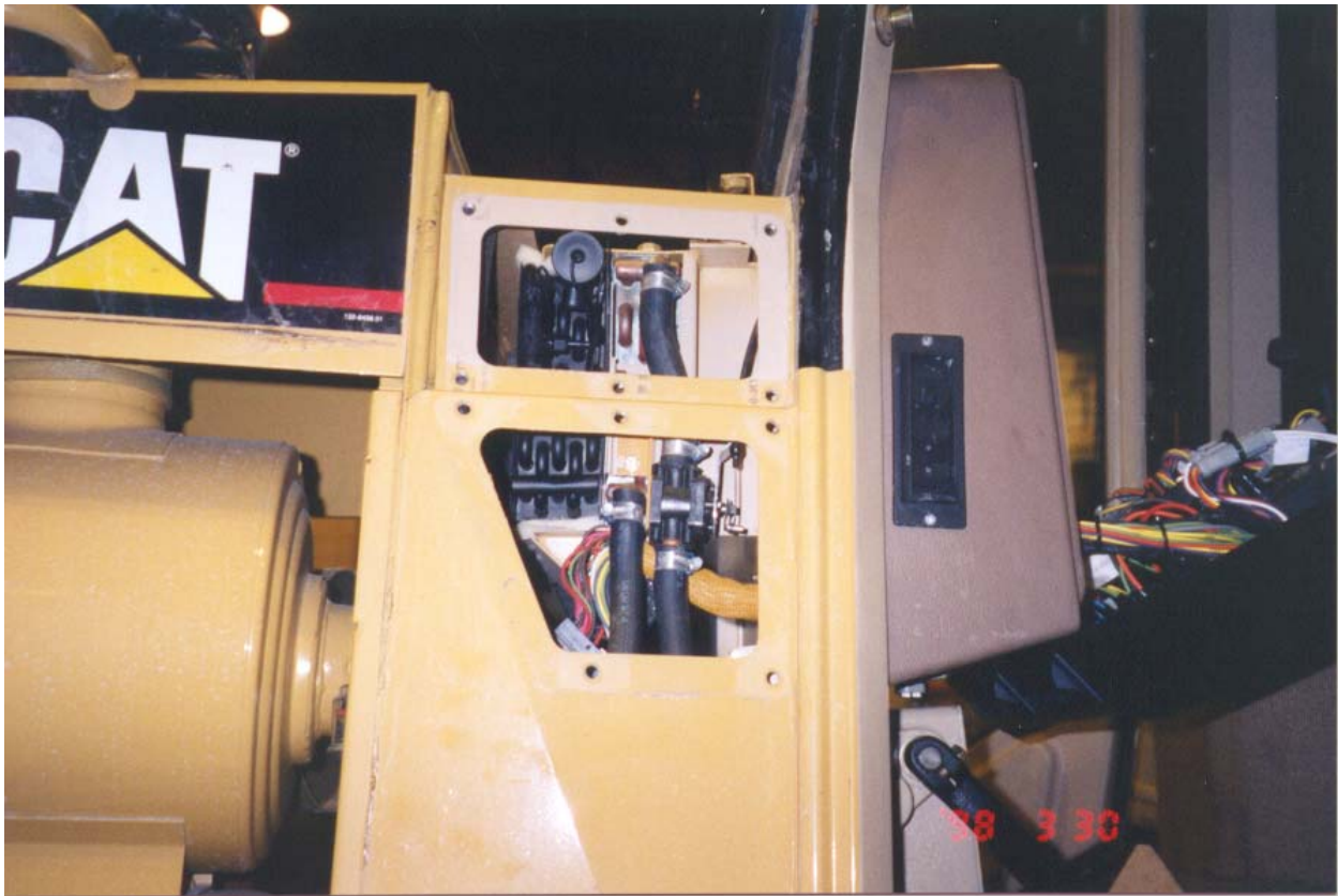
Evaporator in place alongside heater coil.
